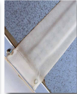
9 Burnish once more to optimize adherence and conformance to uneven surfaces.
