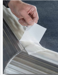
8 Peel off the protective release liner.
